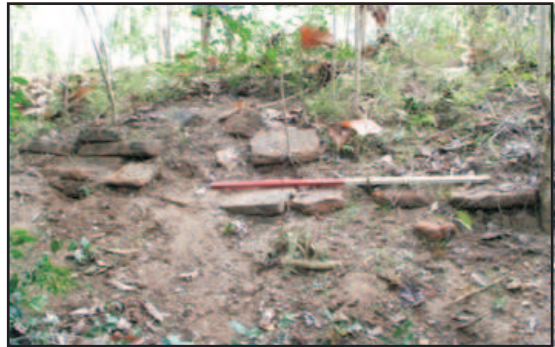
Figure 4. Right bank of canal that commence from Neelabamma dam of Kala Oya
